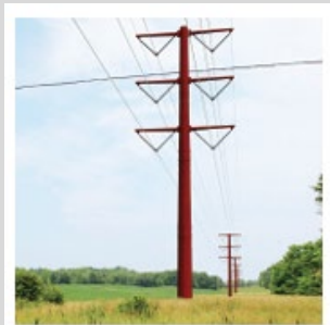
This simulated image demonstrates a 345-kV transmission line 'double-circuited' with a 1150kV transmission line.
