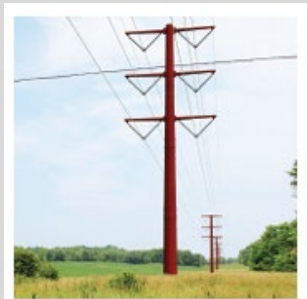
This simulated image demonstrates a 345-kV transmission line 'double-circuited' with a 1150kV transmission line.
